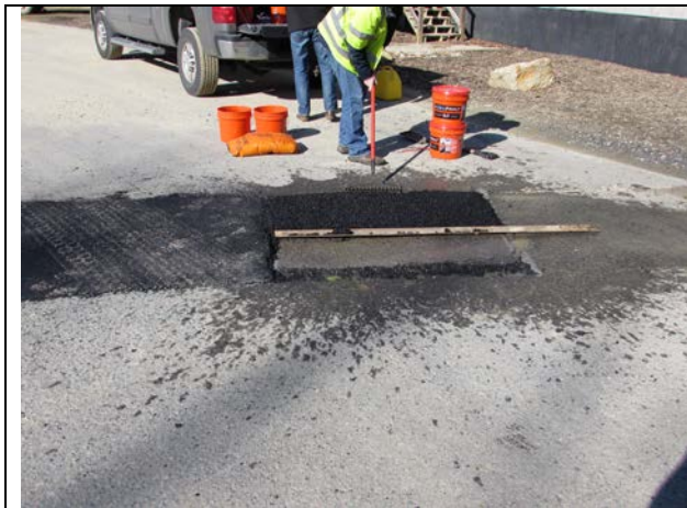
Figure 4. Aquaphalt spread & raked
