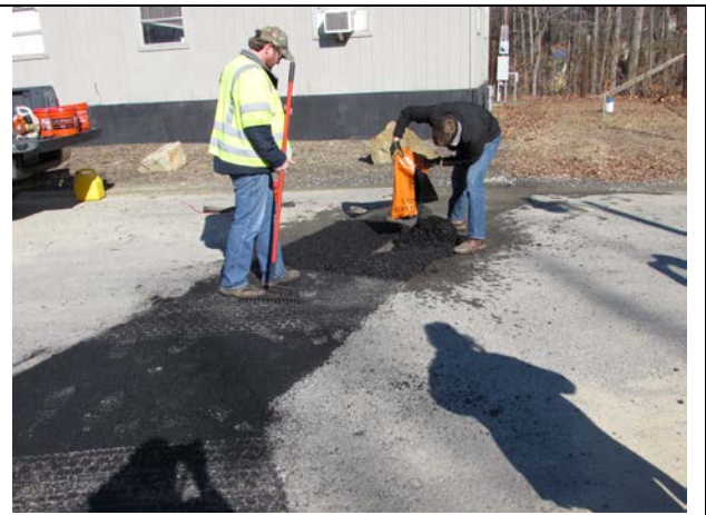
Figure 5. Bond-X spread & raked
