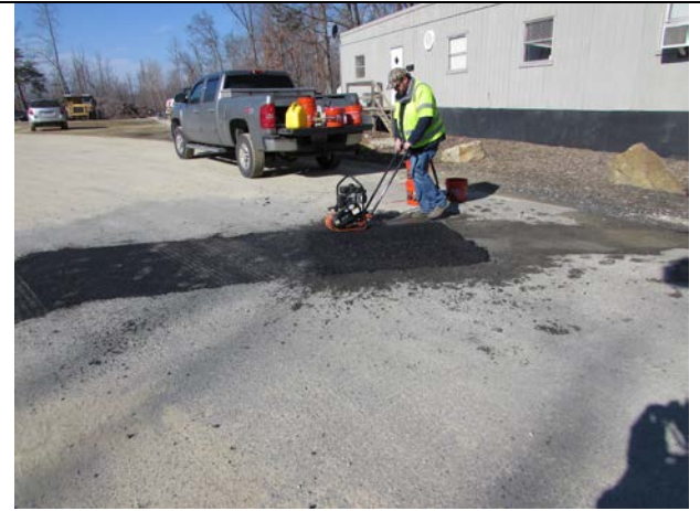
Figure 7. Both Compacted with Flat Plate
