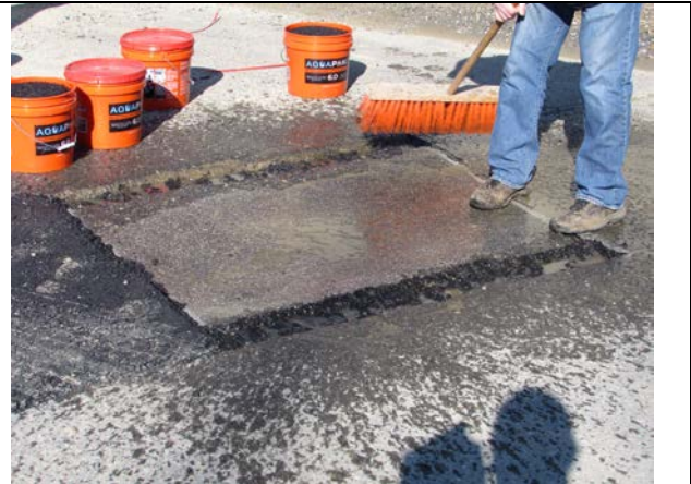
Figure 3. Area cleaned, wetted, & broomed near side Bond-X, far side Aquaphalt
